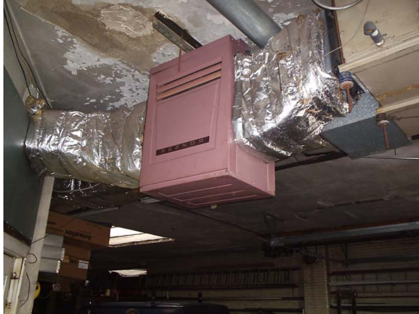
Photograph 7: Overhead Natural Gas Fired Heating Equipment
